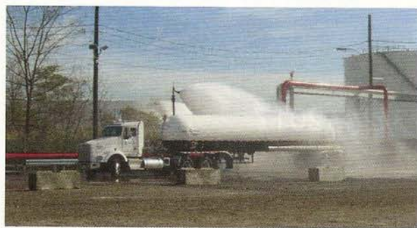
Figure 2. Butane offloading station.
