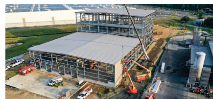
FIG. 1. Project status 18 mos into construction.
