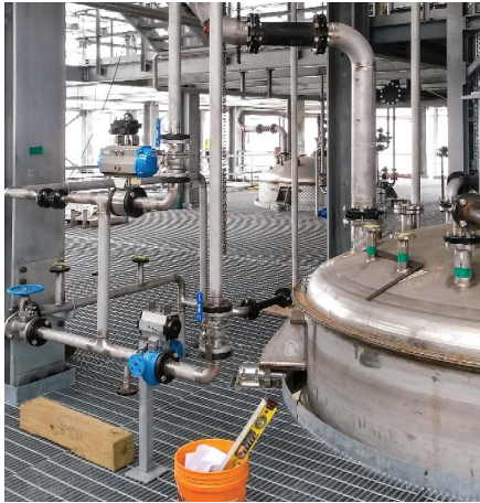
FIG. 3. Project status 18 mos into construction.
