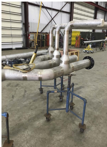
Figure 4. Pipe spool fabrication in shop.
