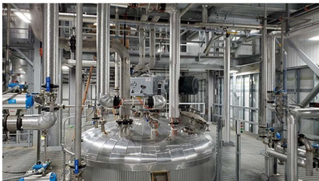
Figure 3. Specialty chemical plant expansion.
