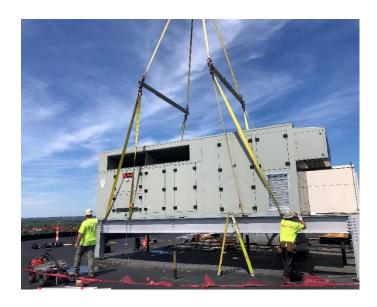
ShureLine Construction replaced a roof top air handling unit in early 2020 at Chester, PA. Working with a general contractor (GC), ShureLine completed the project safely, on budget and on-time. The scope of work included:
