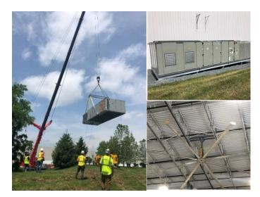
A general contractor (GC) approached ShureLine Construction to help install new air handling units (AHU) in an unconditioned warehouse.
